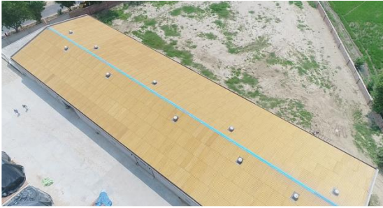
Everest Super Manufacturing Plant, Gidderbaha, Punjab
